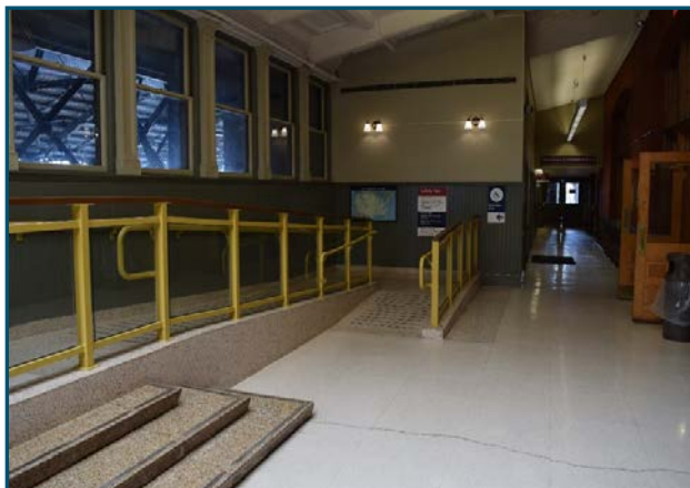
Ramp from main station entrance to passenger waiting area at the station in Harrisburg
