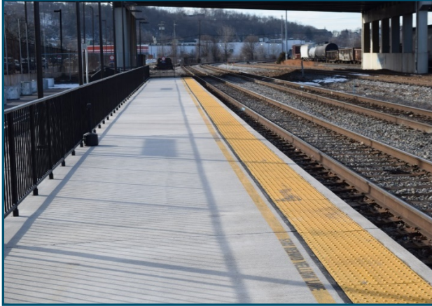
Platform with detectable warning system at the station in Cumberland
