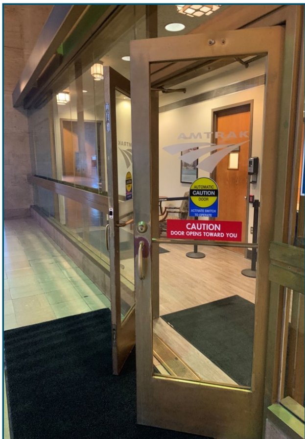
Automatic doors to customer service office at 30th Street Station, Philadelphia
