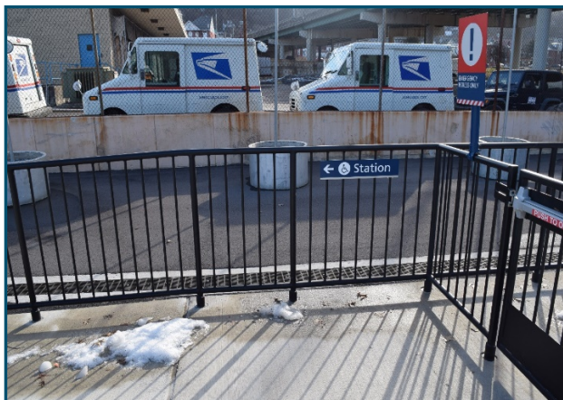
Accessible emergency egress ramp at the station in Cumberland
