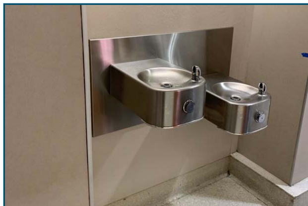
Accessible water fountain at 30th Street Station, Philadelphia
