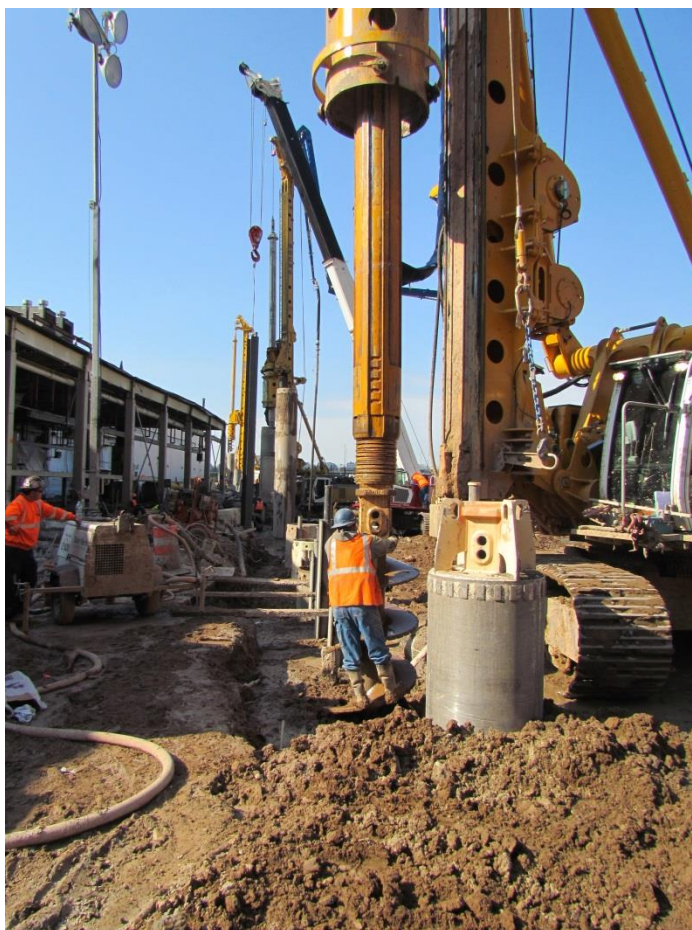
Gateway program’s concrete casing project underway Photo: Amtrak OIG
