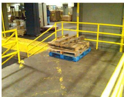
Figure 2. Example of the Removal of a Safety Barrier
