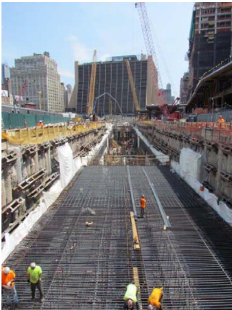
Ongoing construction for the Gateway Program.
