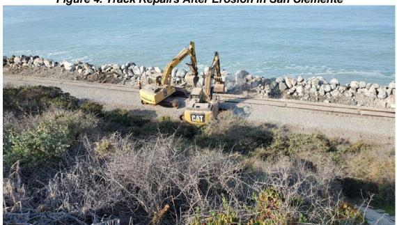
Figure 4. Track Repairs After Erosion in San Clemente
